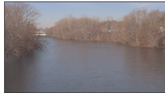
Dundee Dam, river mile 17.4
