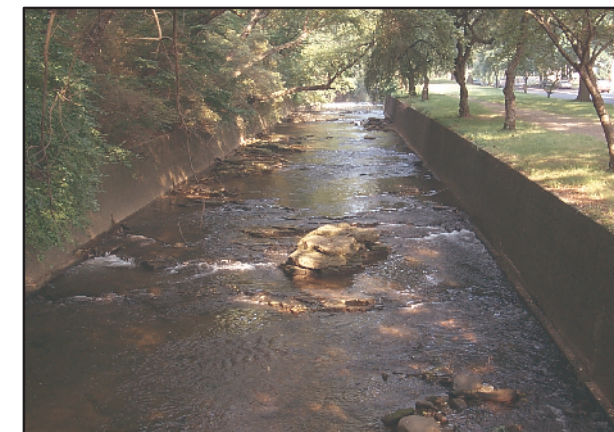
Second River: Looking east in Bellville Park along Mill Street
